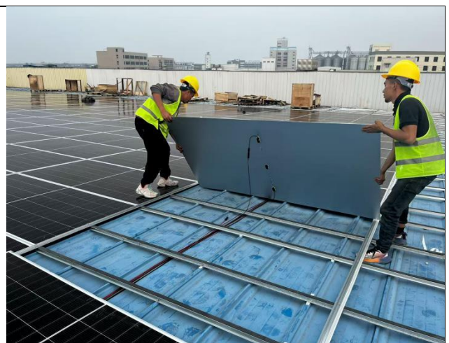
Two workers installing the panel
