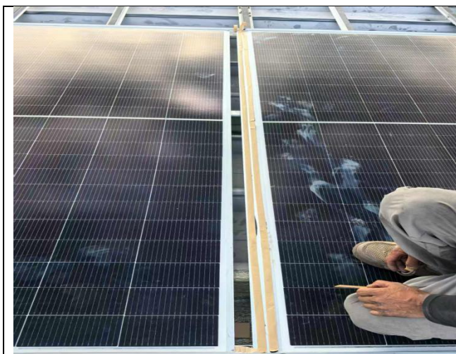
Apply butyl tapes to the upper end of the photovoltaic panel
