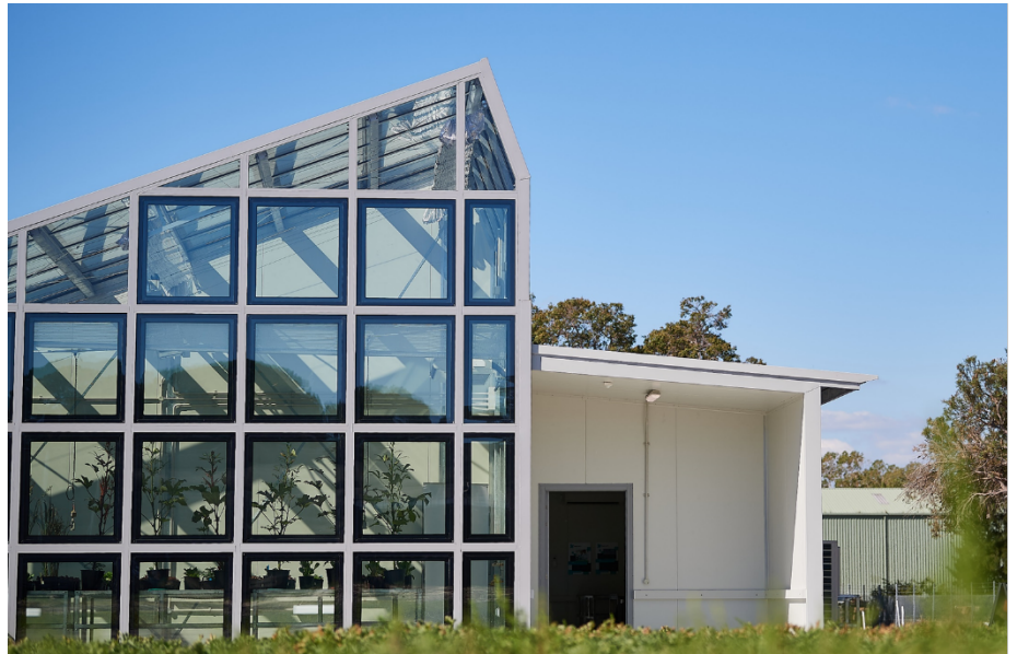
ClearVue's world-first clear solar glass greenhouse at Murdoch University, Western Australia
