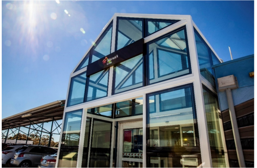
ClearVue's solar glass windows installed at Warwick Grove Shopping Centre, Perth, Western Australia
