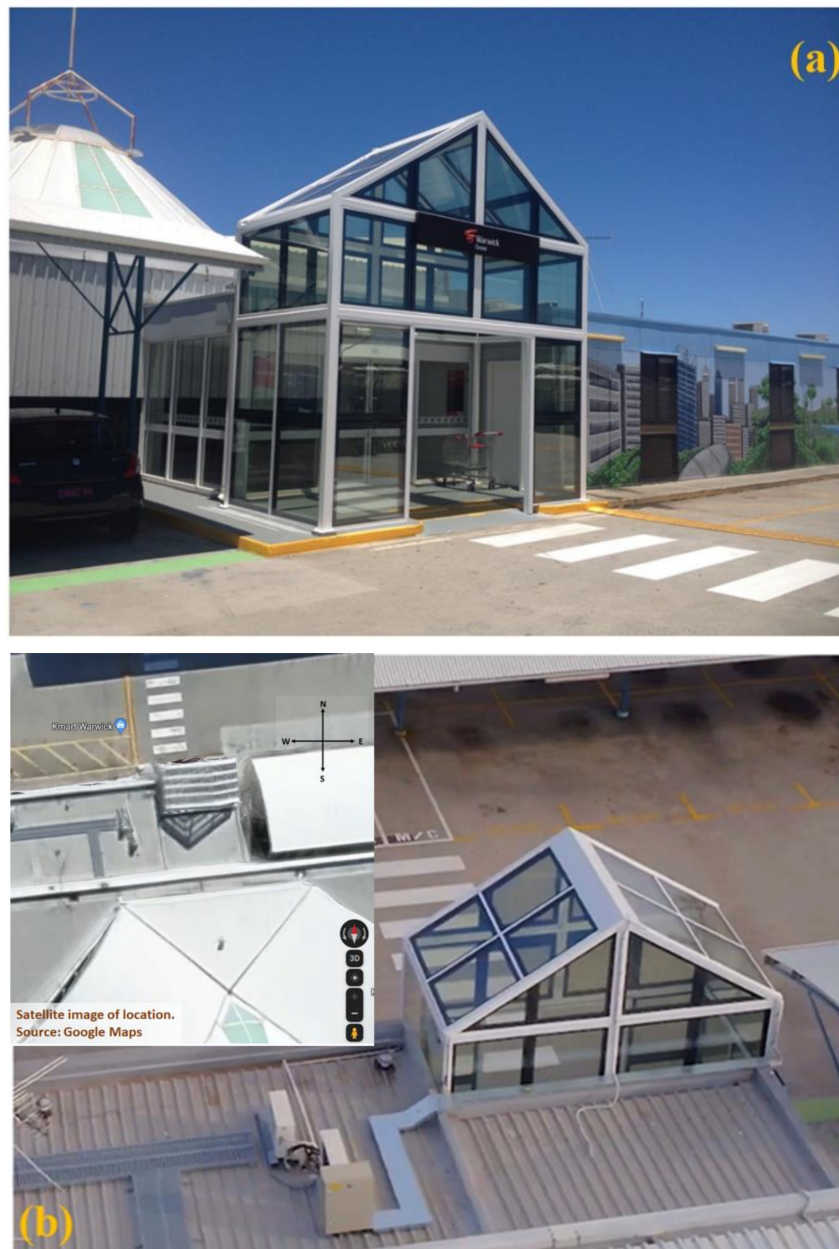
Figure 1. Entrance porch (atrium) of Warwick Grove Shopping Centre in Warwick (Perth, WA, Australia) constructed using 18 solar windows supplied by Clearvue Technologies Ltd. (Perth, WA, Australia). (a) front view and (b) top view, with the inset showing satellite image of the same entrance atrium structure prior to solar windows installation. The site orientation-related data are also shown; the roof sides are tilted at \approx 37^\circ from horizontal plane.
