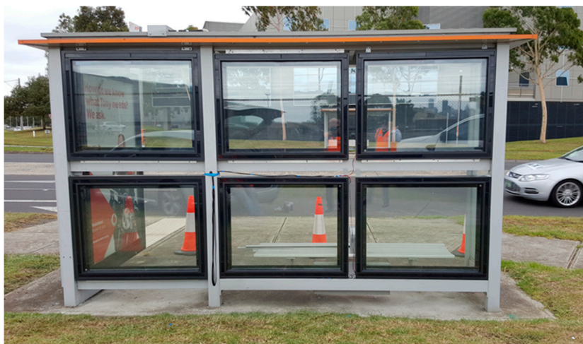
Figure 9. Solar window-powered bus stop installed by Adshel, Inc. (Melbourne, Australia).
