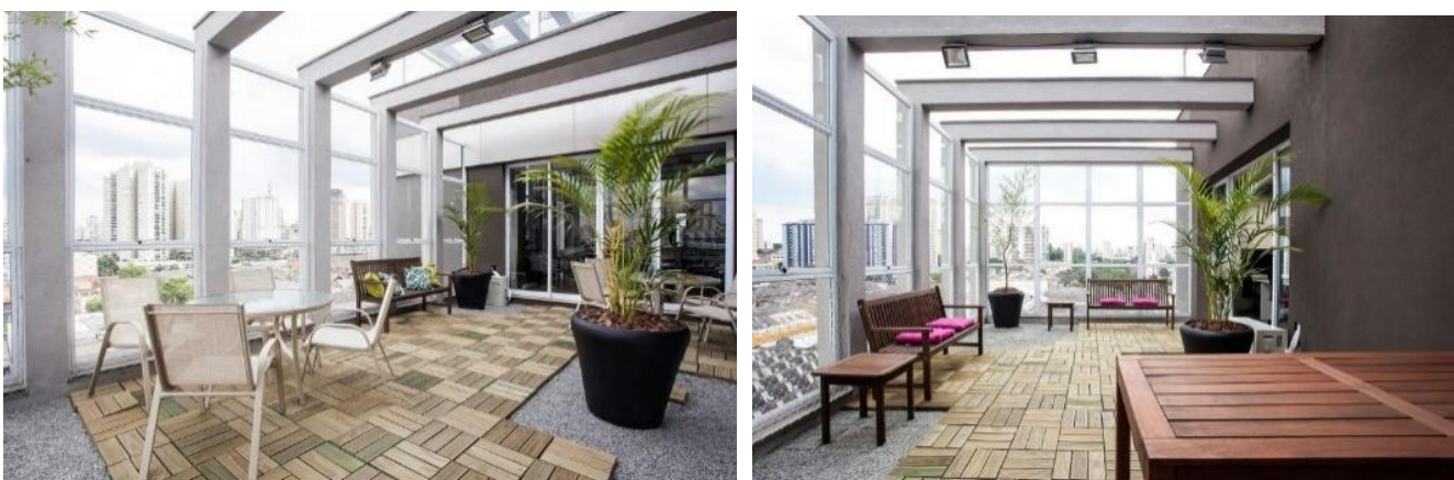
Roof of AMB Brasil's office building to be upgraded with approximately 100m 2 of ClearVue PV solar glazing to be used as a showroom but also for use in completion of INMETRO Brazilian product testing.
