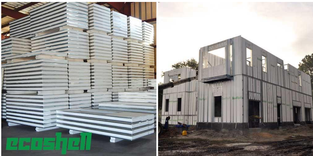
Images of the Insulsteel EcoShell panels in the factory and in a new construction project.
