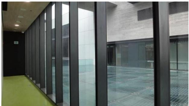
*Recent glazing project completed by Full Treasure at Tuen Mun Siu Lung Government Complex, Area 14 Hong Kong – project used SunnyGlass with Suntuive thermochromic layer by Pleotint USA as an automatic sun-shading solution.*
