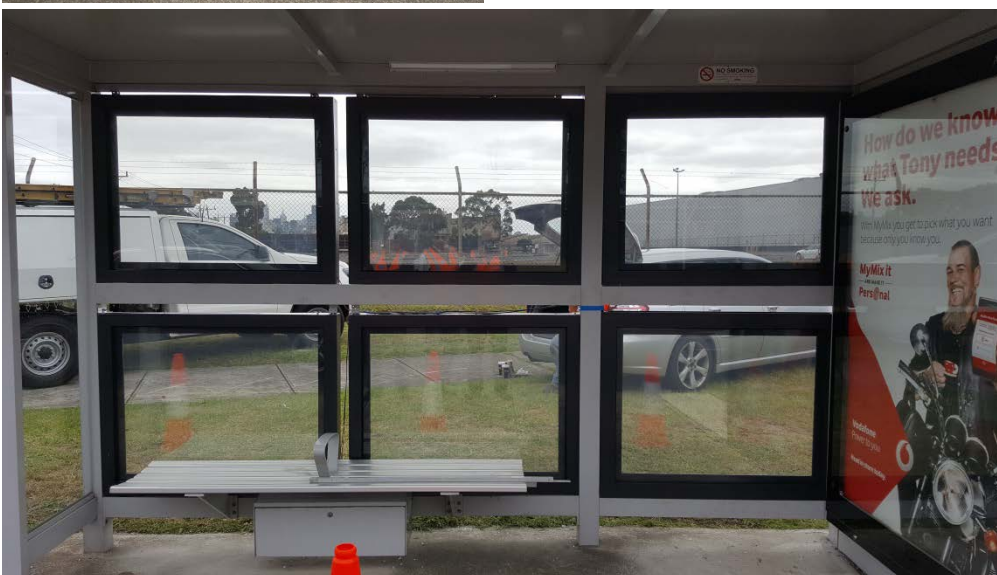
Bus Shelter employing ClearVue panels for powering LED light and Digital Display
