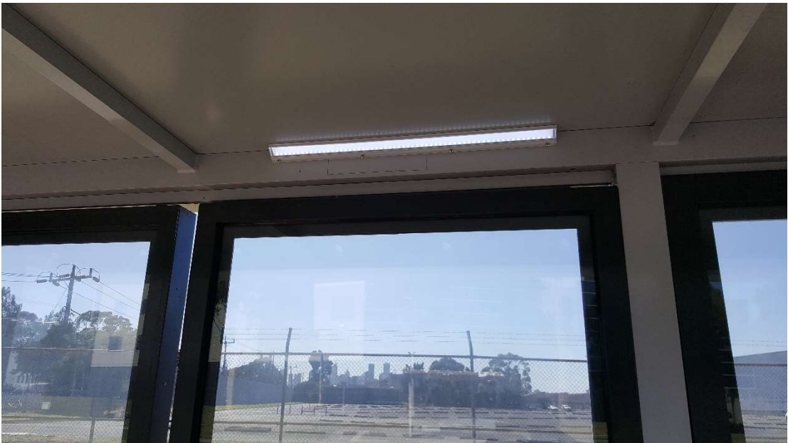
ClearVue Glass powering the Bus shelter light
